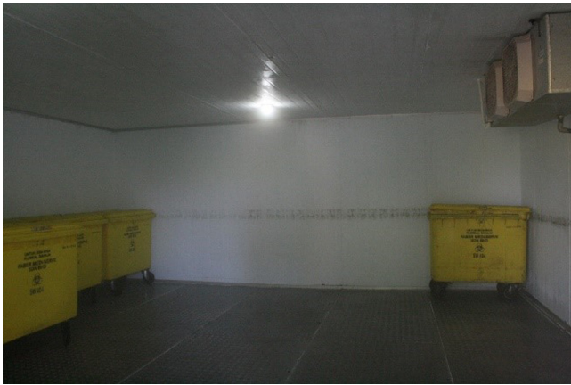
Fig 12. Clinical waste cold room of the hospital before modification.
